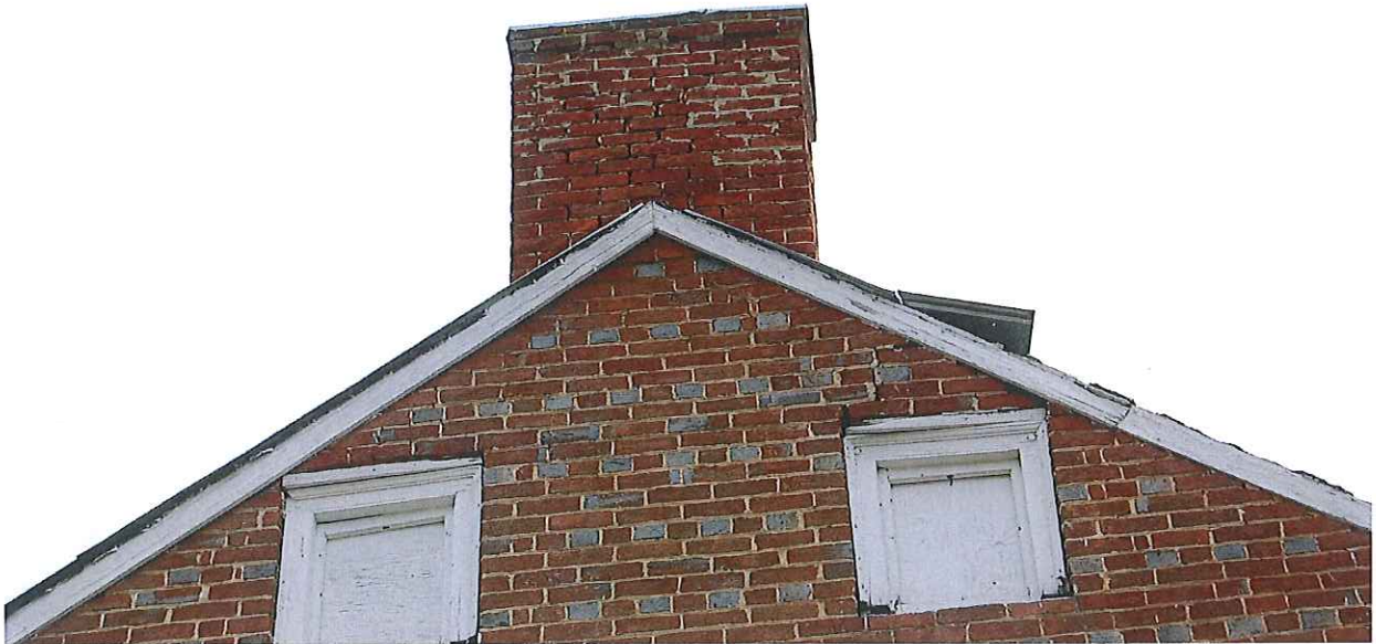
Photo #4: West side chimney detail
