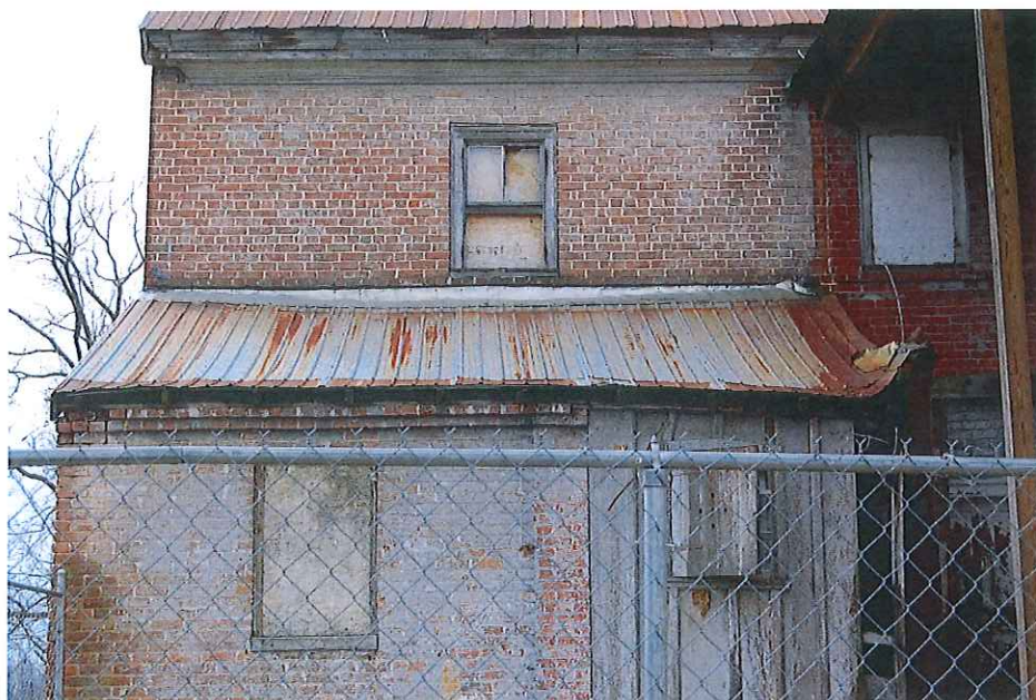
Photo #1: Addition roof, north side
