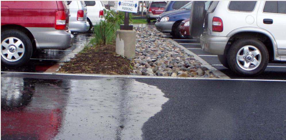
Photo: Harbor Engineering. Note: Standard, impervious pavement is shown on left side of photo under the pooling water. Pervious pavement is shown on right side of photo, where water has absorbed into the pavement. Also note the medians designed to assist with stormwater runoff.
