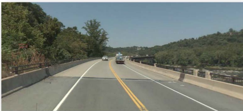
Figure 13: Harpers Ferry Bridge at Shenandoah River, Source: Google Maps
