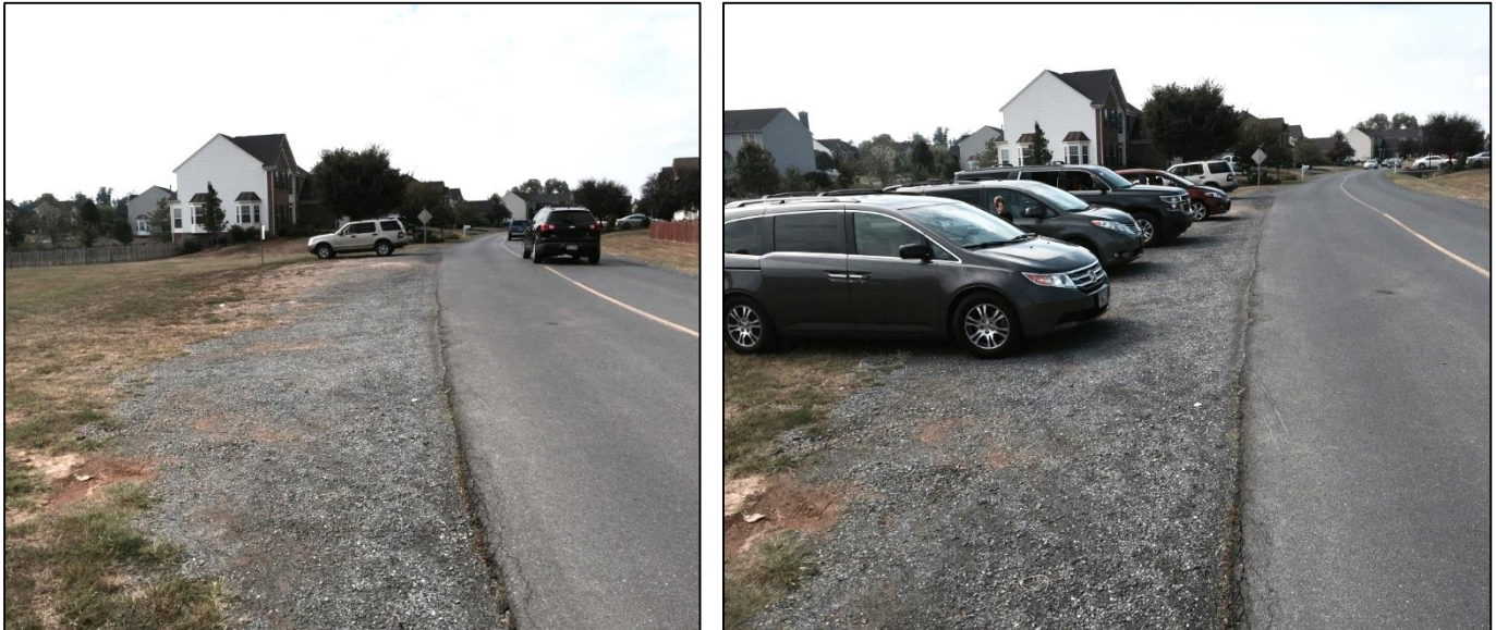
Above: Existing conditions of gravel and dirt pad where parents wait/Vehicles stacked in pad waiting for the bus
