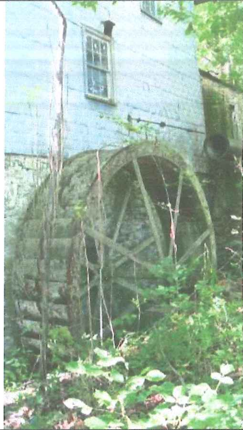
Figure 3. Feagans' Mill from the north showing Fitz Water Wheel manufactured in Martinsburg, West Virginia. WV_Jefferson_County_Feagans'_Mill_0003
