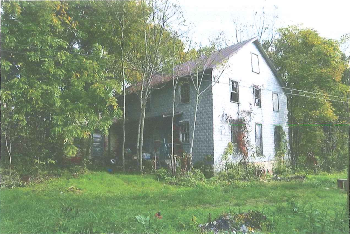
Figure 1. Feagans' Mill from the southwest. WV_Jefferson County_Feagans'_Mill_0001
